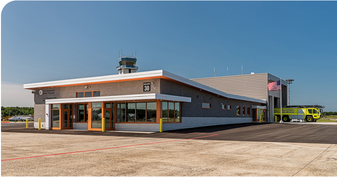
Hanscom Airfield Rescue and Fire Fighting Facility Hanscom Air Force Base, Bedford, MA
